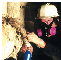
LEAD & ASBESTOS REMEDIATION
