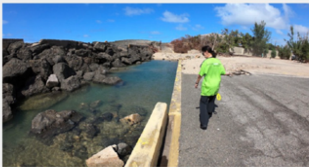
Shown is a Matrix staff member in Puerto Rico during the company's Hurricane Maria Damage Assessment work in 2017. Matrix primarily focuses on environmental, civil infrastructure and engineering.
