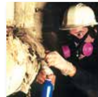
LEAD & ASBESTOS REMEDIATION
